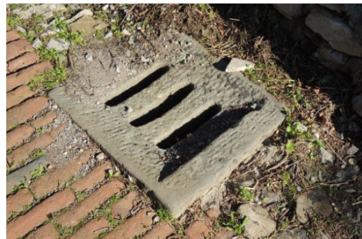
Fig.5. Sandstone storm drain (Source: Fabio Fratini).
