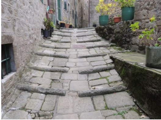
Fig. 1. Traditional sandstone paving in the village of Stiappa (Pistoia Apennines-Tuscany) (credits Fabio Fratini).
