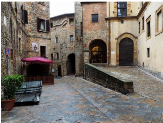
Fig. 2. Traditional paving made of Pietra Panchina in Volterra (Tuscany) (Source: Fabio Fratini).
