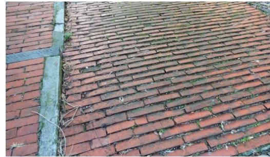
Fig.7. New, smooth bricks on which a thin biological patina is forming (Source: Fratini).
