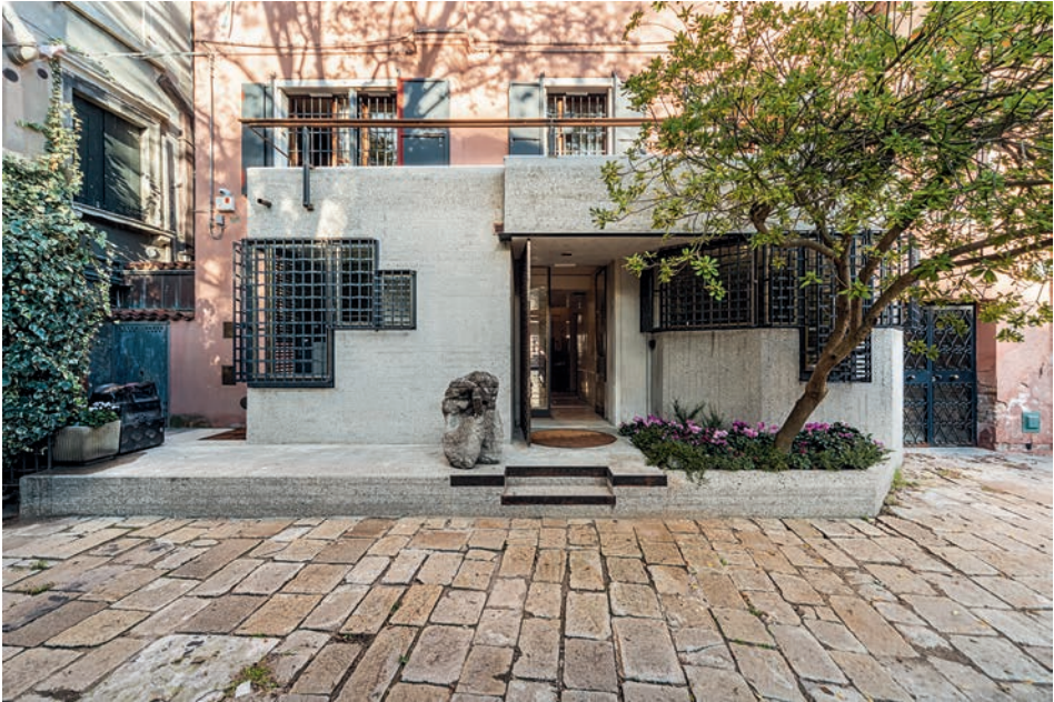
fig. 1. Casa Balboni, view of the facade towards the garden after restoration. (© Claudia Rossini)
