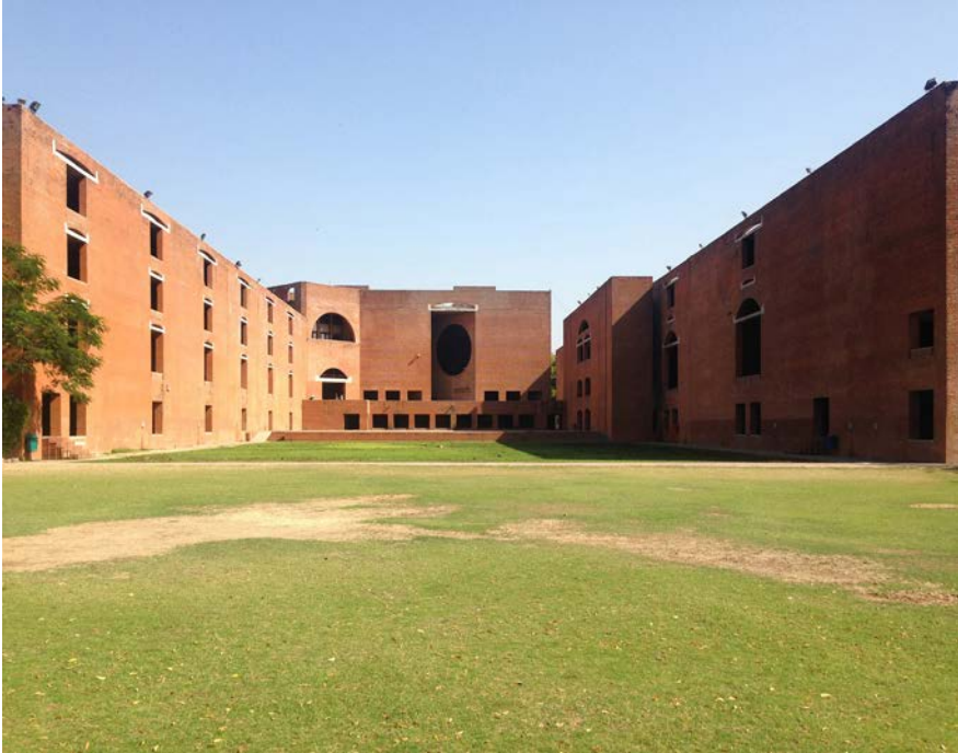
fig. 1. IIMA, Ahmedabad, Main Complex and Louis I. Kahn Plaza. (© Alessandra Rampazzo, 2015)
