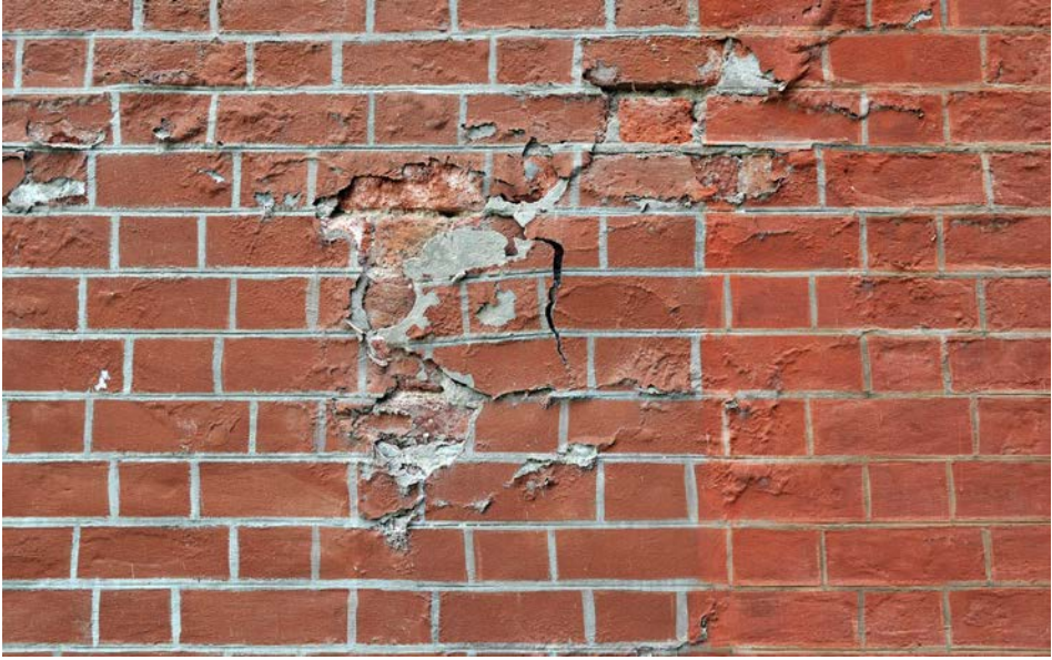
fig. 2. IIMA, Ahmedabad, Main Complex: the covering and the simulation of the brickwork as a pictorial work. (© Alessandra Rampazzo, 2015)
