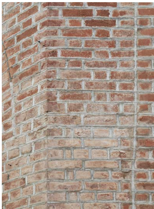
fig. 3. IIMA, Ahmedabad, Dorm D12: change on the used bond. The picture shows the English bond in the lower part and the flemish bond in the upper one. (© Alessandra Rampazzo, 2015)
