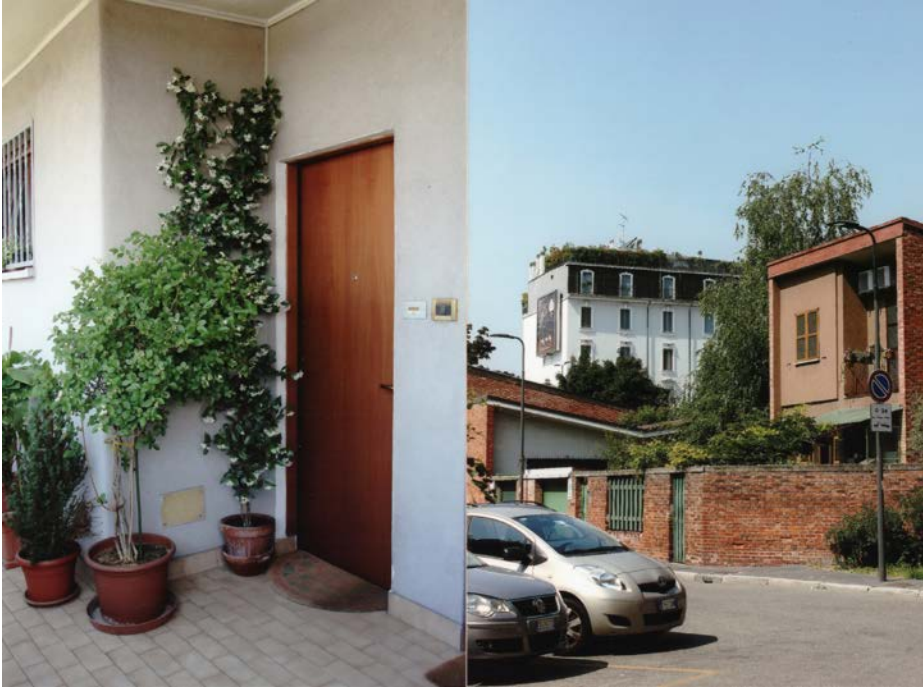
fig. 3. INA-Casa Neighborhood Harar-Dessiè, Milan, 1951-1955. Building Via Harar 3, G. Ponti, L. Ghò: entrance from the balcony / Insulae Via Val Pantena 7, L. Figini, G. Pollini. (Photo sequence from the photoworkshop Everyday Architectural Heritage, © Architectural Preservation Studio – A. Canziani 2017, AUIC School, Politecnico di Milano)
