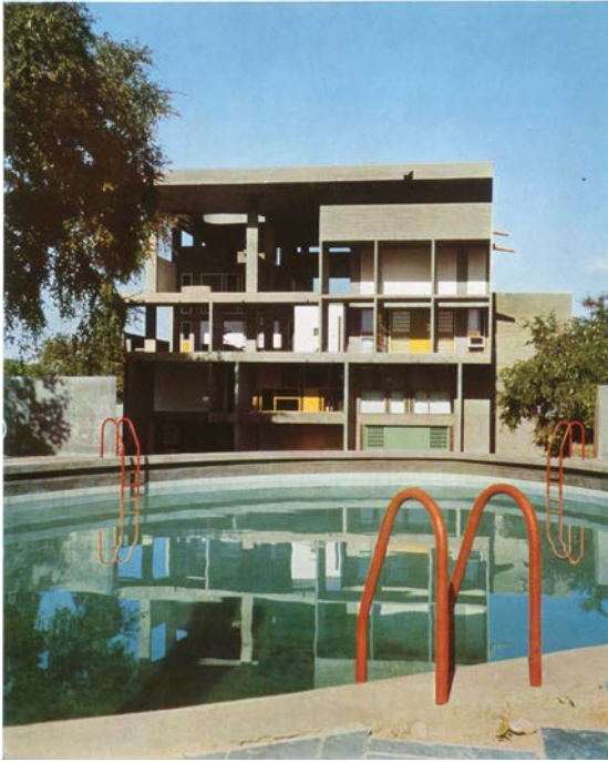
fig. 1. Villa Hutheesing-Shodhan, Ahmedabad, India, 1951- 56, south-west elevation. (© Fondation Le Corbusier / SIAE)
