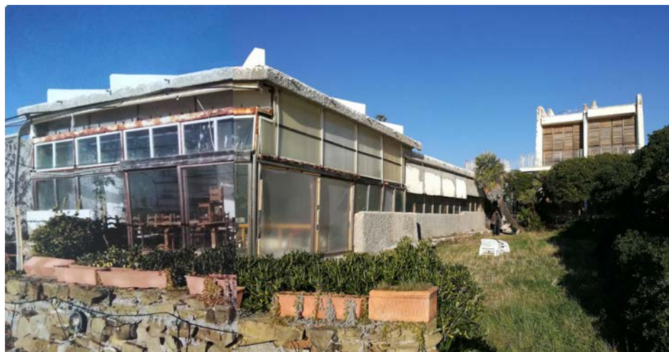
fig. 2. Fig. 2 Villa La Saracena before the restoration works, 2016. (© Paolo Verdeschi)
