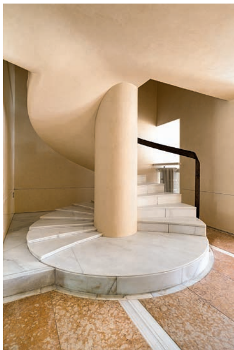
fig. 3. Casa Balboni, the helical staircase after restoration. (© Claudia Rossini)
