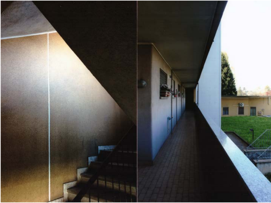
fig. 2. INA-Casa Neighborhood Harar-Dessiè, Milan, 1951-1955. Building Via Harar 3, G. Ponti, L. Ghò: staircase/distribution balcony. Photo sequence from the photoworkshop Everyday Architectural Heritage, © Architectural Preservation Studio – A. Canziani (2017), AUIC School, Politecnico di Milano
