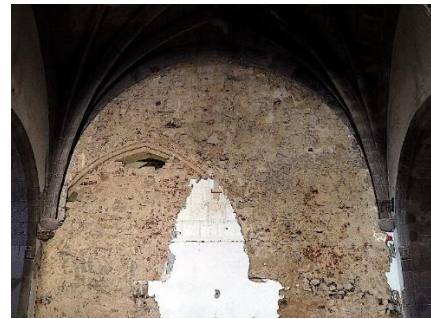
Figure 6. Presbytery post removal with opening
