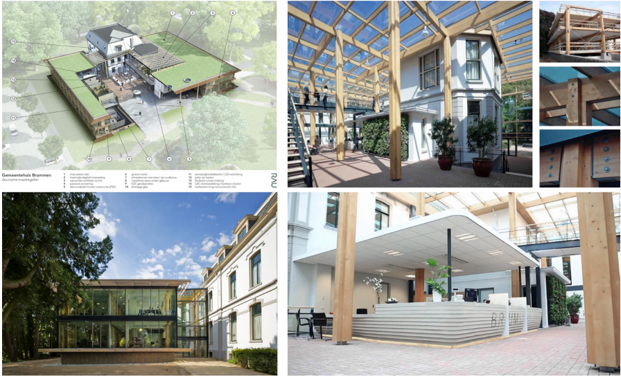
Fig. 10.4 - Temporary City Hall in Brummen, The Netherlands, designed in 2013 by RAU Architects with reversible technologies that turn it into a raw material depot for future buildings' applications (Source: www.rau.eu)
