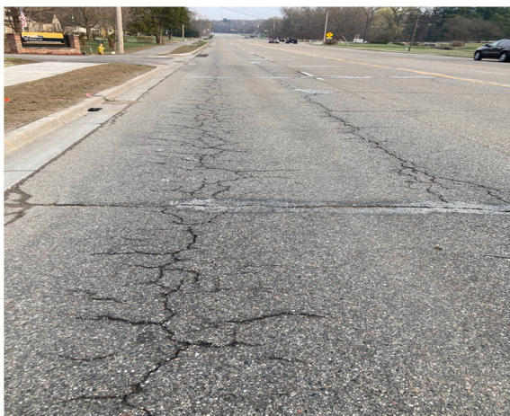
(a) Original Pavement Condition
