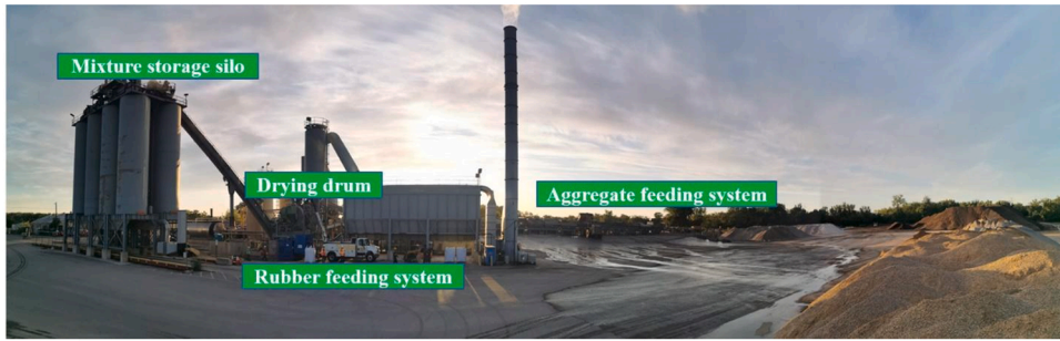
Fig. 4. Asphalt plant applied to supply the GTR-modified HMA and the polymer-modified HMA.
