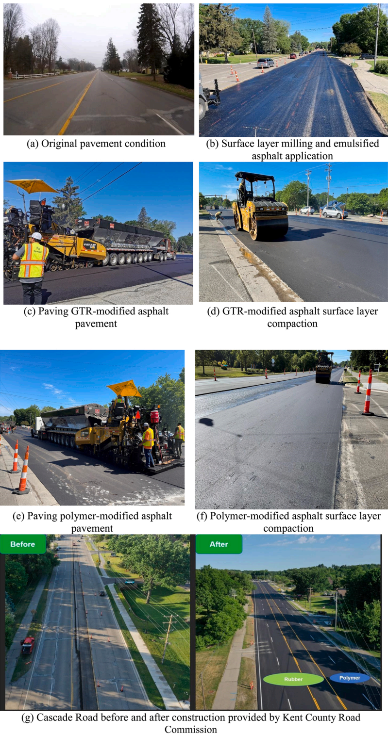
Fig. 12. Pavement construction procedure on the Kent project.
