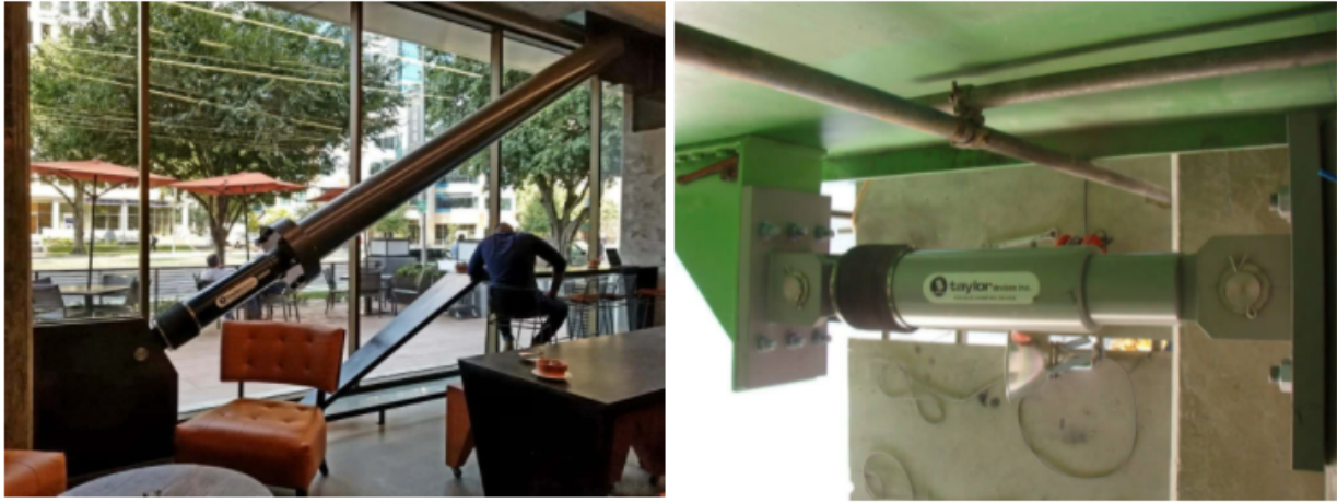
Figure 1.2. Fluid viscous damper. Source: Taylor Devices Inc. (Tay, 2022).
