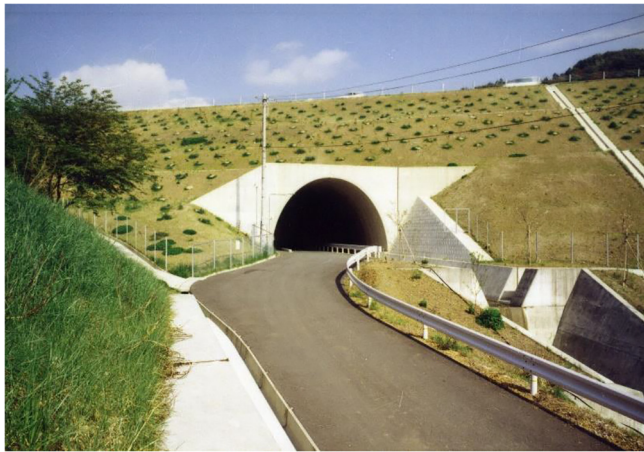
Fig. 4. Field situation of constructed three-hinge precast arch culvert.
