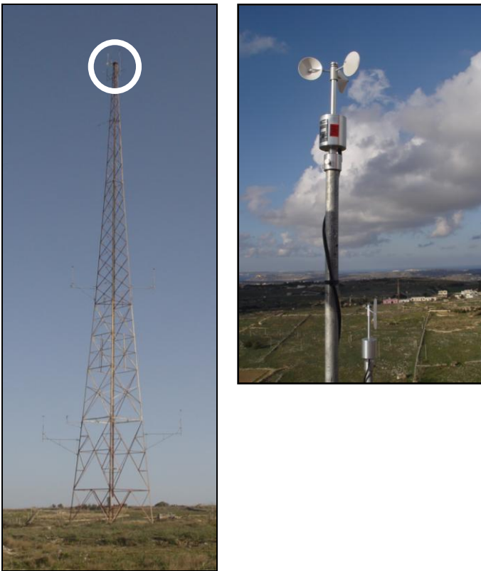
Figure 2: The left-hand photo shows the 45 metre former telecommunications tower being used for wind monitoring purposes at Wied Rini (Site A). The right hand photo shows a close-up of the anemometer and wind direction vane at the topmost mast level.
