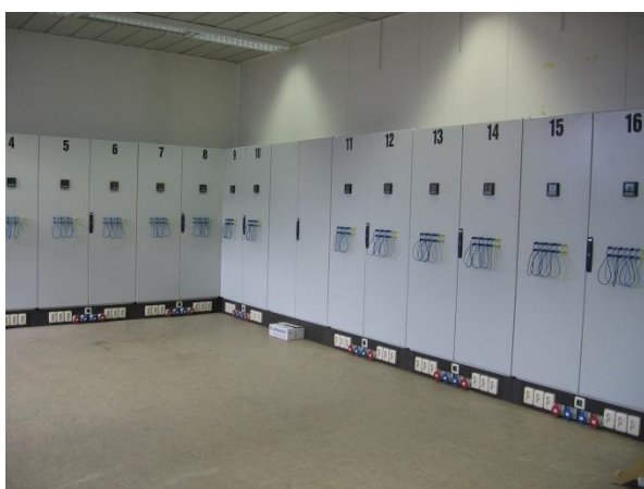
Fig. 5: general overview of the actual test facility
