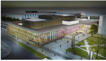
Fig. 1.16 Maastricht Exhibition and Conference Centre (MECC) Maastricht, Netherlands.
