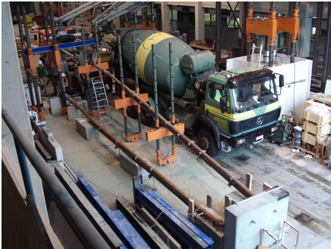
Figure 3: Loop circuit with a length of 25 m.
