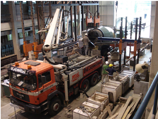
Figure 2: Truck mounted concrete piston pump.
