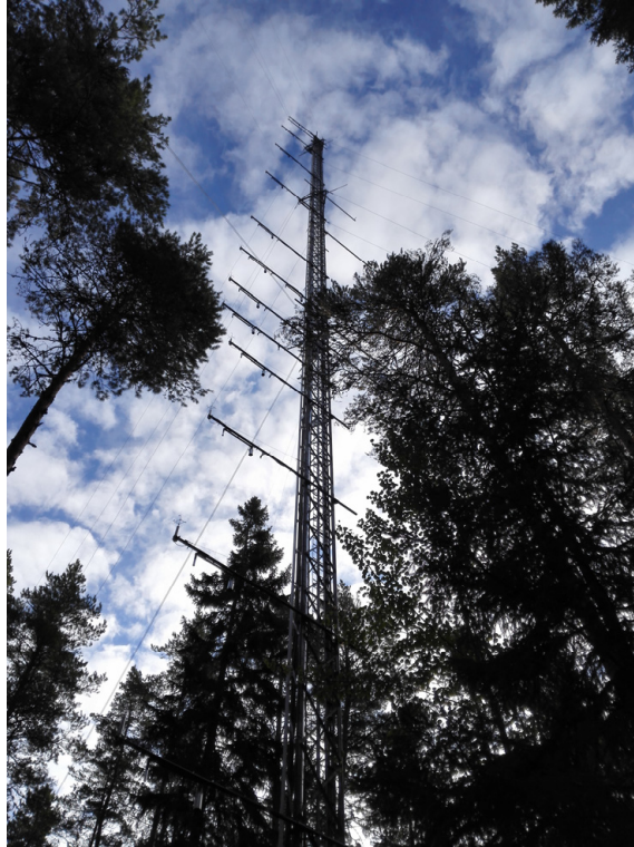
Figure 1. The eddy covariance tower at the Norunda site. Photograph: Sofia Junttila
