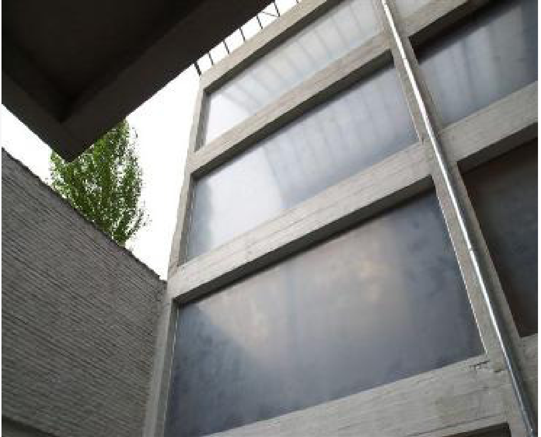
Figure 49: Gallery Jan Colle, Belgium.
