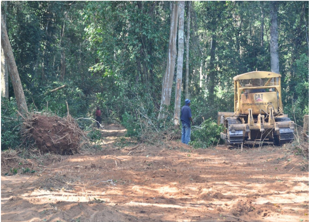
Photo 1: Trees along the narrow public road being cleared for road expansion in Zaraninge forest reserve in SANAPA
