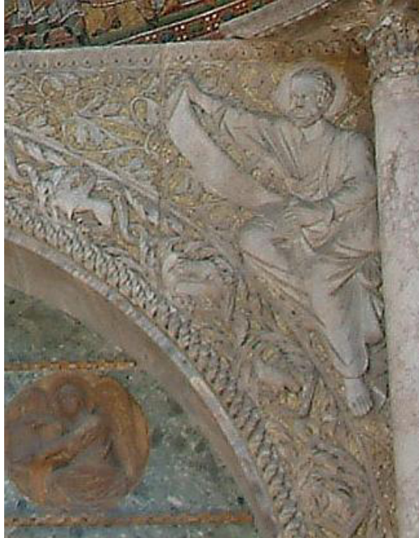
Figure 1.4: Illustration of a spandrel. Close-up of one of the spandrels of San Marco's Cathedral in Venice (Italy). The spandrel results as an architectural by-product from fitting a dome upon rounded arches, and was later filled with biblical scenarios. Picture from Wikimedia Commons.
