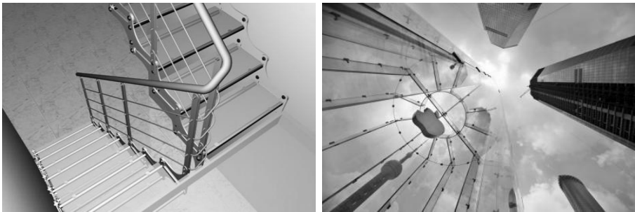
Figure I.1: Structural glass applications: staircase with four-sided supported glass treads (left); high-end full-glass structure (Apple store, Bohlin Cywinski Jackson architects, 2010, Shanghai) (right)
