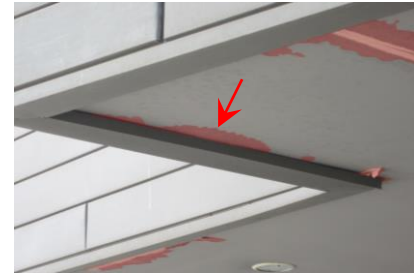
Figure 3. Moisture stains.
