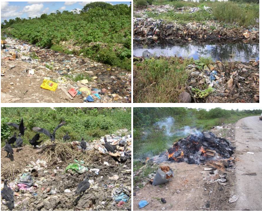
Photo 3.5: Effects of inadequate operation at the dump: the drainage ditches are full of plastics; black birds (vultures) are attracted by organic waste, burning of waste
