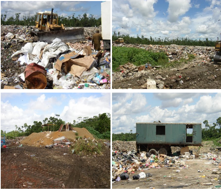
Photo 3.3: Open dump Ornamibo Facilities at the dump: bulldozer to spread the waste, sand to cover the waste (sometimes), shelter for the workers
