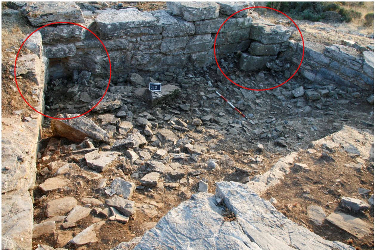
Fig. 8. The two drainage channels of Cistern no.1 (2010). Picture taken from the northeast.
