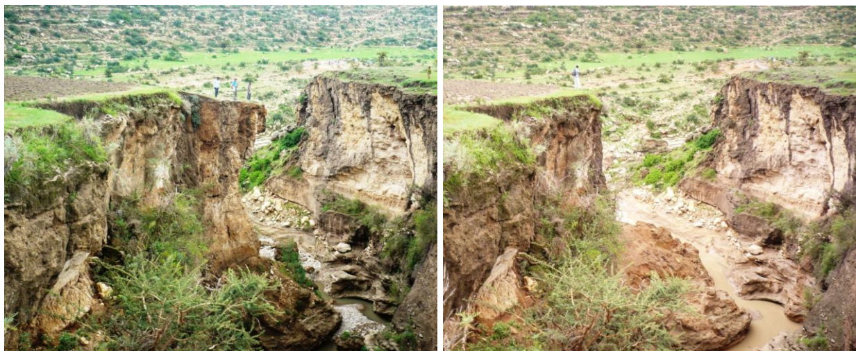
Fig. 5. Gully sidewall erosion by a large slab failure was caused by undercutting and the development of tension cracks parallel to the gully wall. Photographs by A. Frankl before (left) and after (right) an important rainfall event in the summer of 2010, when flood marks rose up to 3.5 m in the main gully (Fig. 6).
