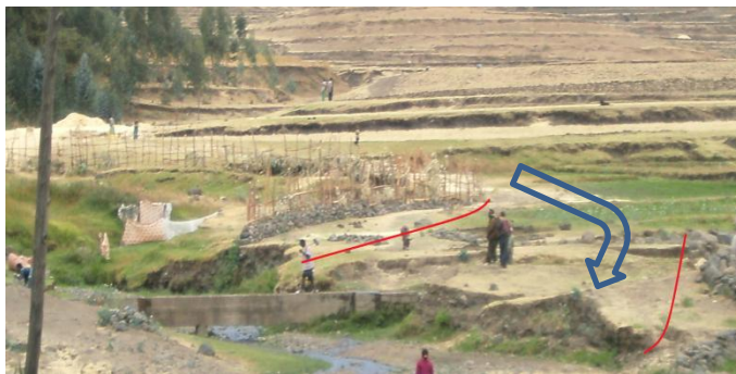
Figure 8: Location with red arrow of the silted gullies in Atsela (left; 12.93180°N – 39.52446°E) and Sinkata (right; 14.04785°N – 39.58263°E). The filled blue arrows show the direction of channel diversion for Atsela, and the location of the large gabions for Sinkata. Closer view of the channels in Atsela (lower left) and Sinkata (lower right). The red lines indicate the channel boundaries and the blue open arrow indicates the historical stream direction.
