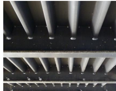
Fig. 5. Orthotropic deck plate of the Temse bridge
