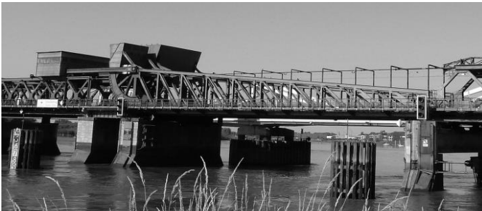
Fig. 4. The Temse bridge across the river Scheldt (Belgium)
