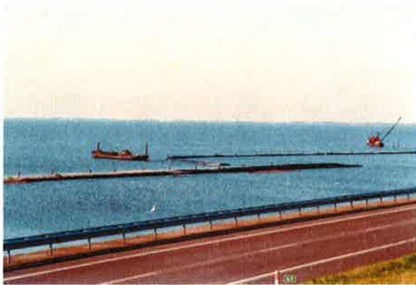
Figure 10. Moment in the construction of secondary dam
