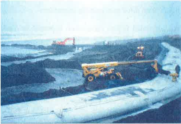
Figure 19. Geotube on the beach
