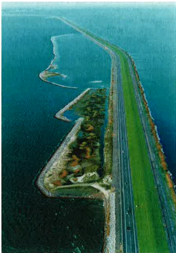
Figure 11. Secondary dam constructed with geosynthetic tubes as a core
