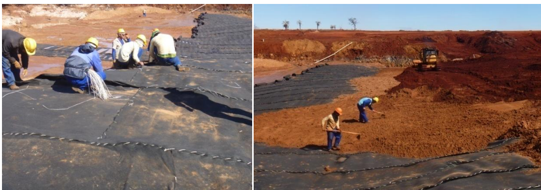
Figure 8 – Placement of geocomposite.
