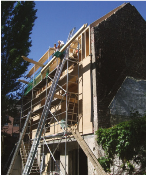
Case Schaarbeek (LCBuild): Deep retrofit of single family house with box-in-box renovation scenario up to high energy efficient building.
