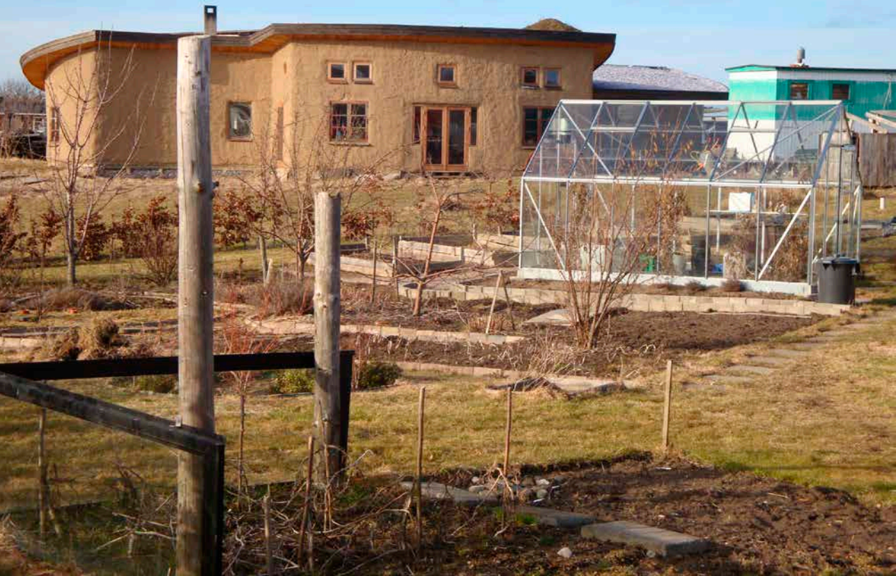
FIGURE 6.5 A sustainable life style and ongoing building activities in Fri og Fro
