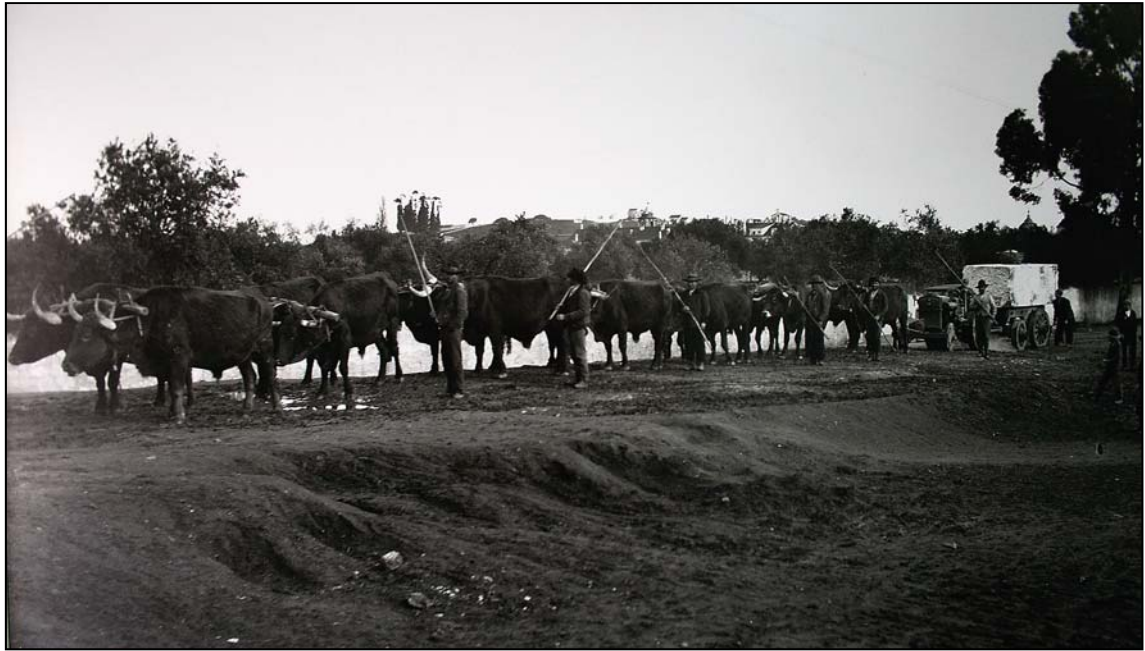
Figure 8.21 Early 20th century CE stone transport in the Estremoz Anticline (Portugal) using seven teams of two oxen harnessed in the same span and combined by with small tractor (Photo owned by Solubema, Sociedade Luso-Belga de Mármore, Bencatel, Portugal).
