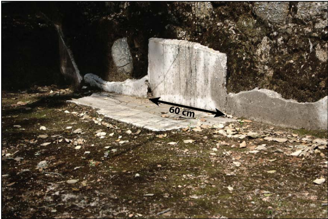
Figure 4.23 Veneer panels in white marble for the wall and floor decoration of the pool in ambiente A .
