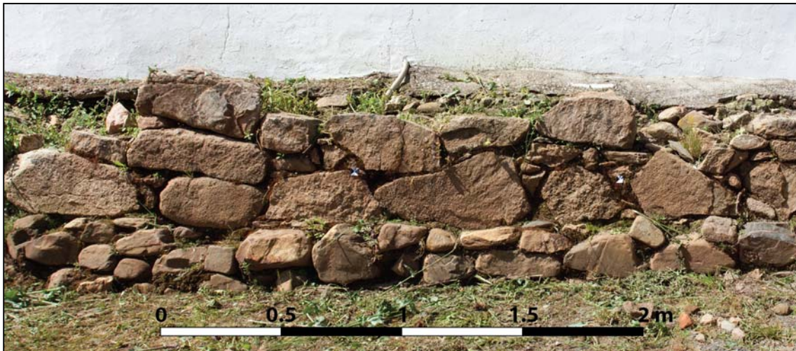
Figure 4.39 Town wall and part of its foundation reused as the foundation for the façade of the Quinta do Deão farmhouse.
