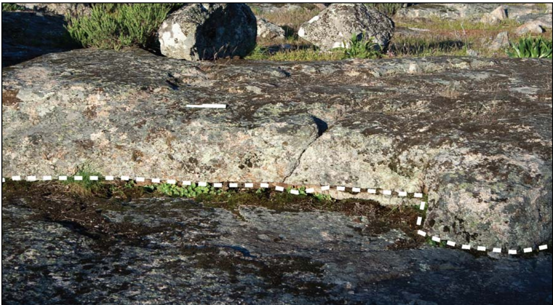
Figure 8.16 Unloading or exfoliation joints exploited for producing granite slabs (scale: 20 cm) (location: 39.368788° N, 7.312846° W (WGS84)).
