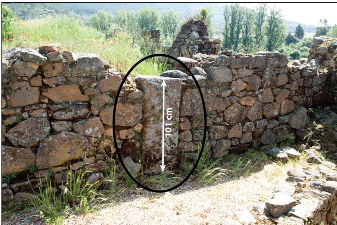
Figure 4.32 Late Roman wall of the South Gate complex characterised by a coarser construction technique and the reuse of granite ashlars from an earlier phase.
