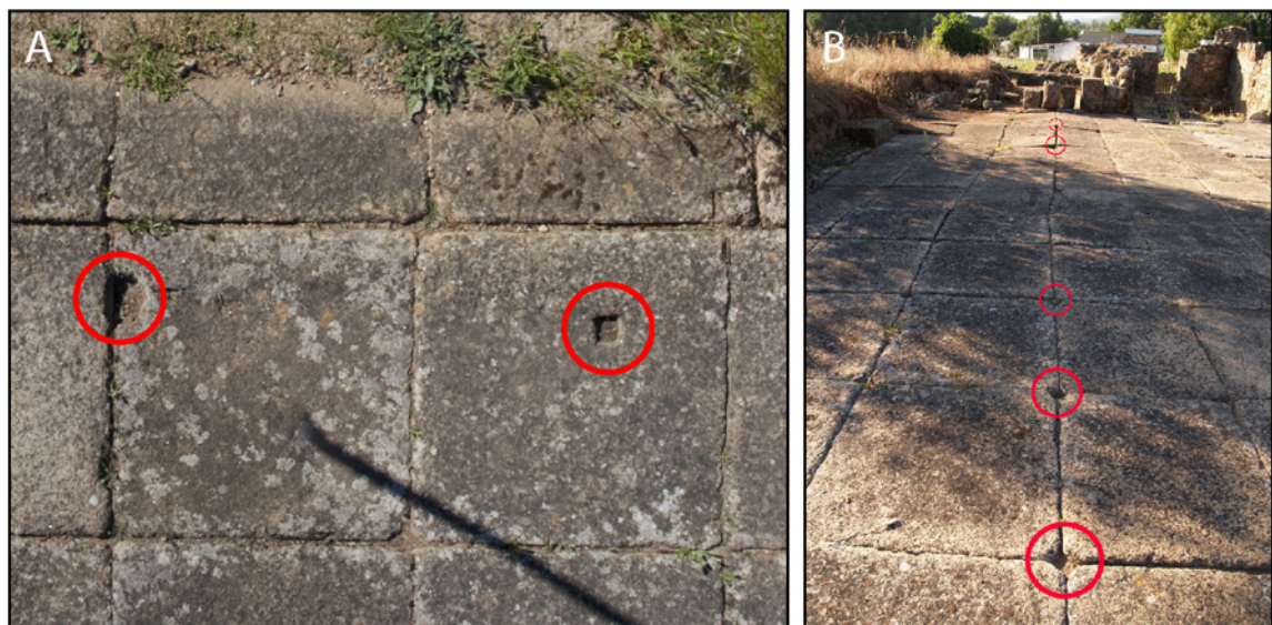
Figure 4.28 (A) Holes for vertical dowels in the northern part of the eastern part of the square; (B) Holes for wooden or iron posts. The square paving blocks measure 88–90 cm. Photo-B by M. Klein.
