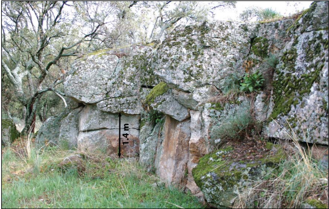
Figure 7.7 Quarry front in the Santo António das Areias quarry with clearly visible natural joints (location: 39.410939° N, 7.351032° W (WGS84)).
