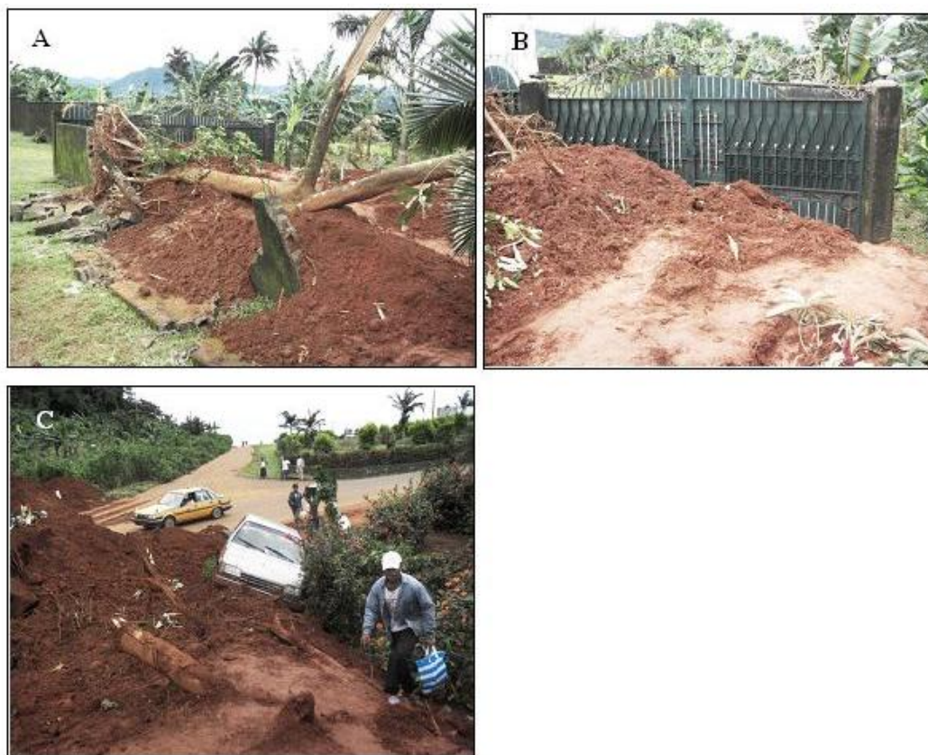
Fig. 2. 24. Typical landslide damage at Kie village; A, B) house destroyed by debris from the 2009 slide at Kie; C) road blocked and vehicle partially buried by slide debris.
