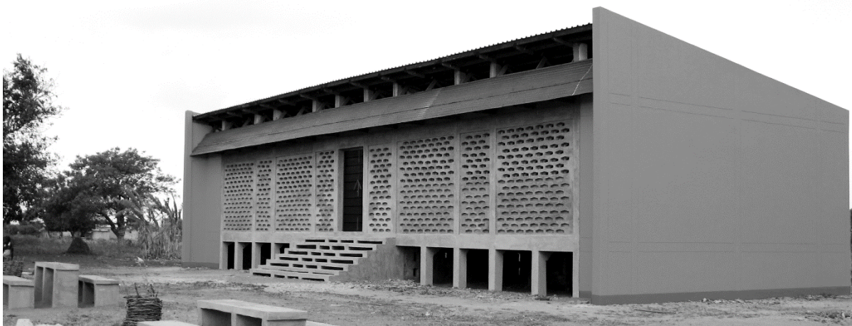
Figure 4.9: Elevated school of Maniquenique, Gaza Province, Mozambique
