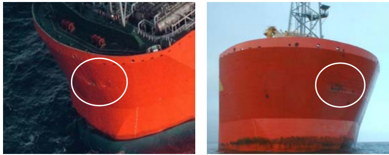
Figure 2-7: Bow indentation due to slamming at the Shiehallion FPSO [13]
