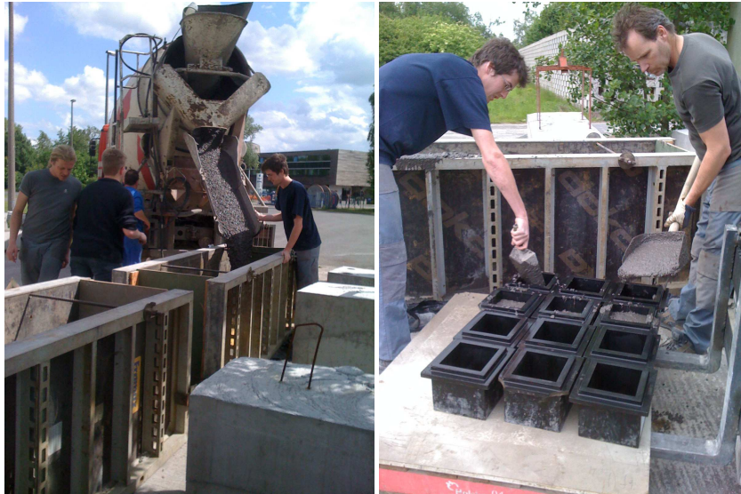
Figure 9.4: Casting SCC in a prismatic formwork (left) and making cubic test samples (right)
