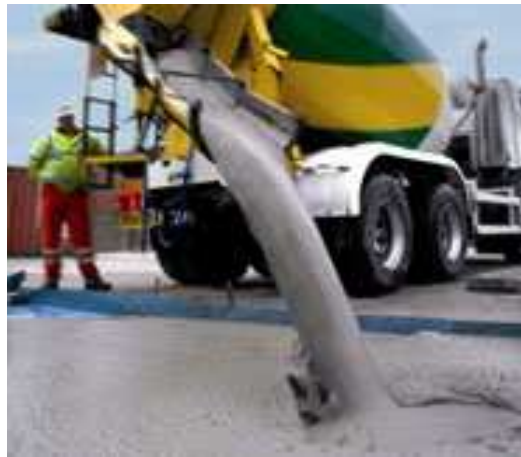
Figure 5.7: Casting of SCC with a good flowing ability
