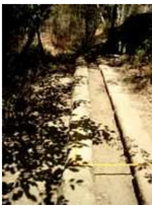
Figure 17: The Roman specus of the western aqueduct discovered in 2004 – detail
