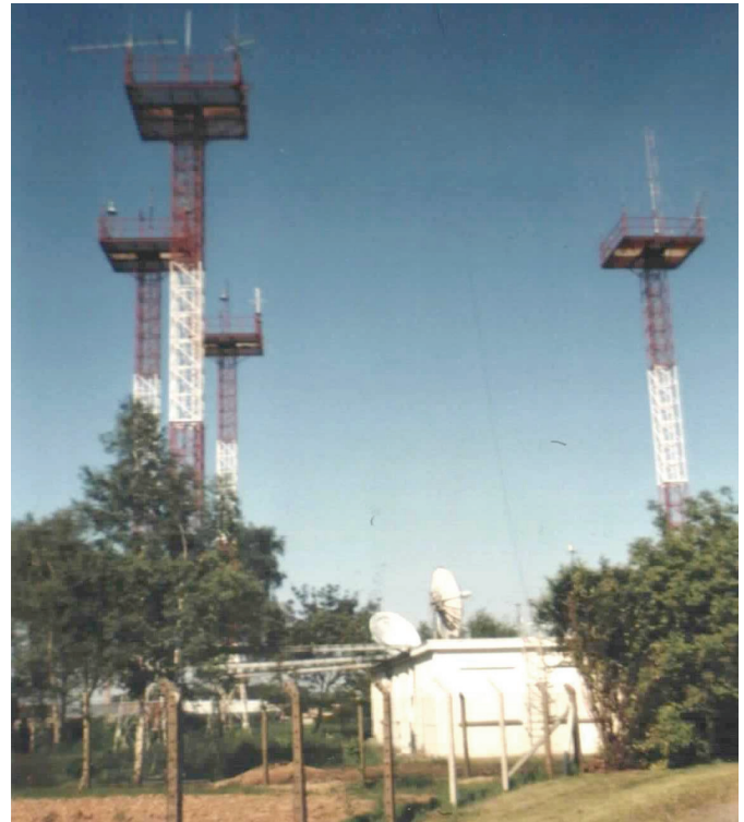
Fig. 1: Reception centre for air to ground communications.
