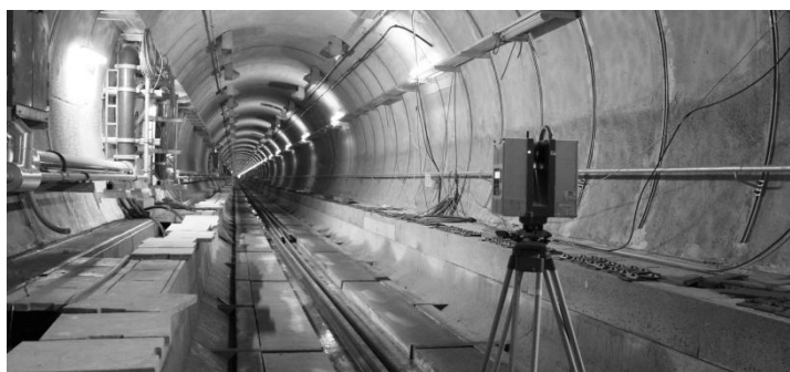
Figure 3 Laser scanner setup
