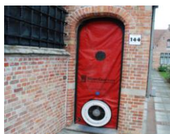
Figure 3 Blowerdoor test to measure the air tightness
