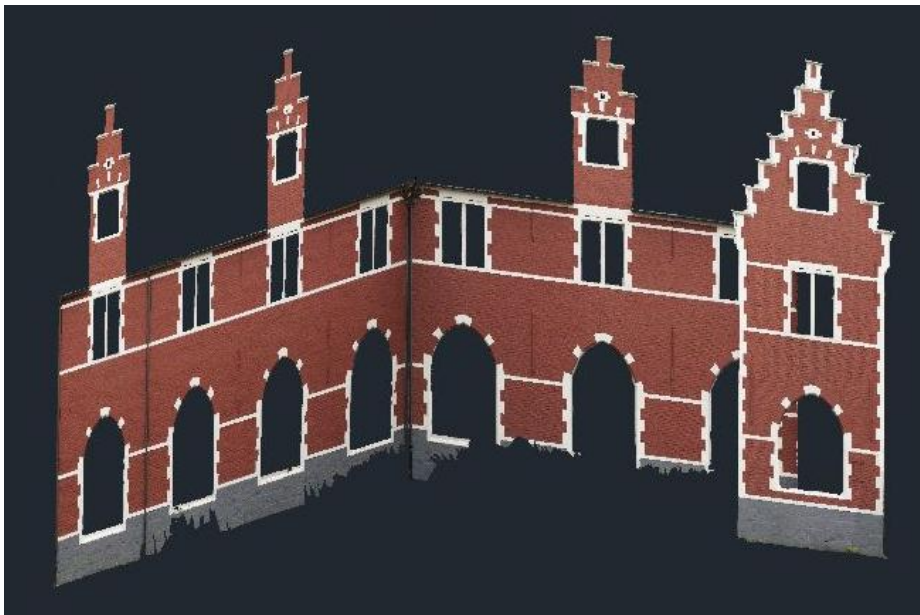
Figure 2: Visualising the orthofoto's of the façades of the Ghent city museum
