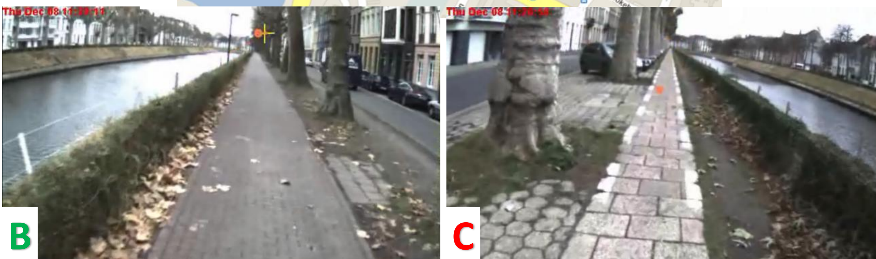
Figure 2 : the cycling route (A) included two bicycle tracks with approximately the same width and similar environment but with different surfaces. The High Quality track (B) was recently renovated and had a brick surface; the Low Quality track (C) had a surface of large tiles that showed several deformities and cracks. Both tracks were physically separated from the carriageway by trees and/or parked cars.
