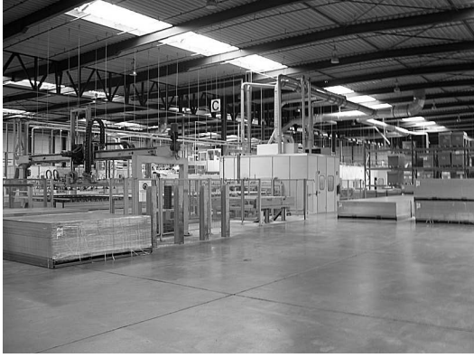
Fig. 1. Measurement environment: production room in a wood processing facility
