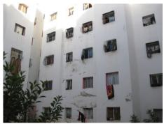
Humidity stains on the outside where the bathrooms are located (May 2010)
