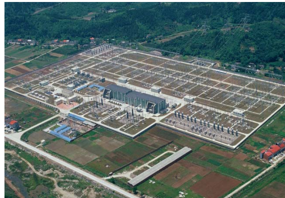
Figuur 4: HVDC omvormer [ABB]
