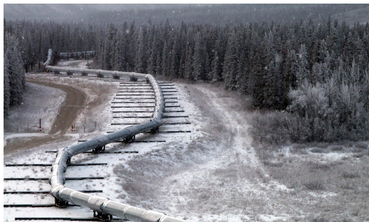
Part of the Trans-Alaska Pipeline System, which survived a Richter magnitude 7.9 earthquake on November 3, 2002 [1.1].
