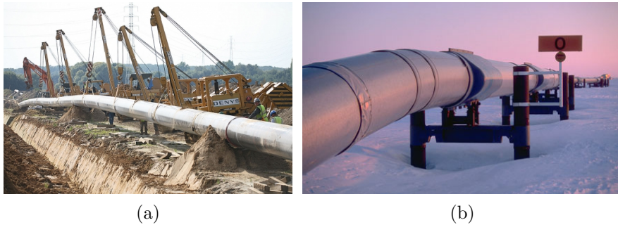
Figure 1.9: (a) Laying of buried pipeline (Source: Denys) [1.23]. (b) Onshore pipeline which operates above ground (Source: Guardian; Photograph: Doug Wilson/Corbis) [1.24].
