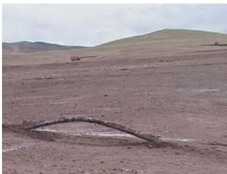
Figure 1.21: Example of frost heaving, observed in the Golmud-Lhasa pipeline [1.65].
