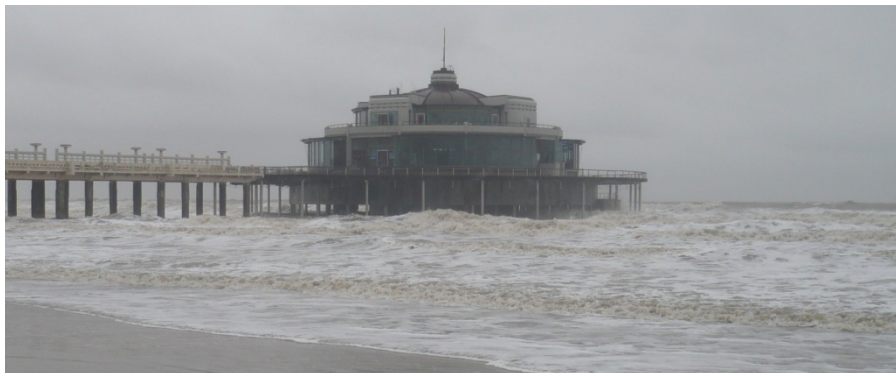
Figure 1.2 The renovated Pier of Blankenberge, Belgium. Picture taken during high tide
