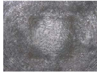
Fig. 15 - Detail of the zone where a concentrated load was applied
