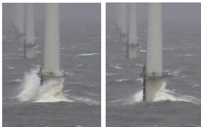
Figure 5-1: Wave run-up on one of the towers of the Horns Rev wind mill farm; H_s = 2.5\text{m} , platform level = 9m above SWL; © Elsam .
