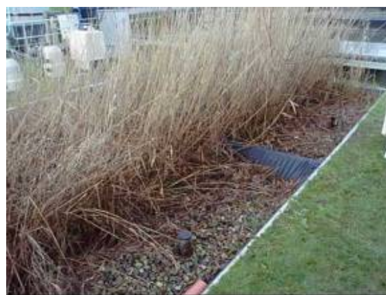
Figure 4.2. Horizontal subsurface-flow reed beds
