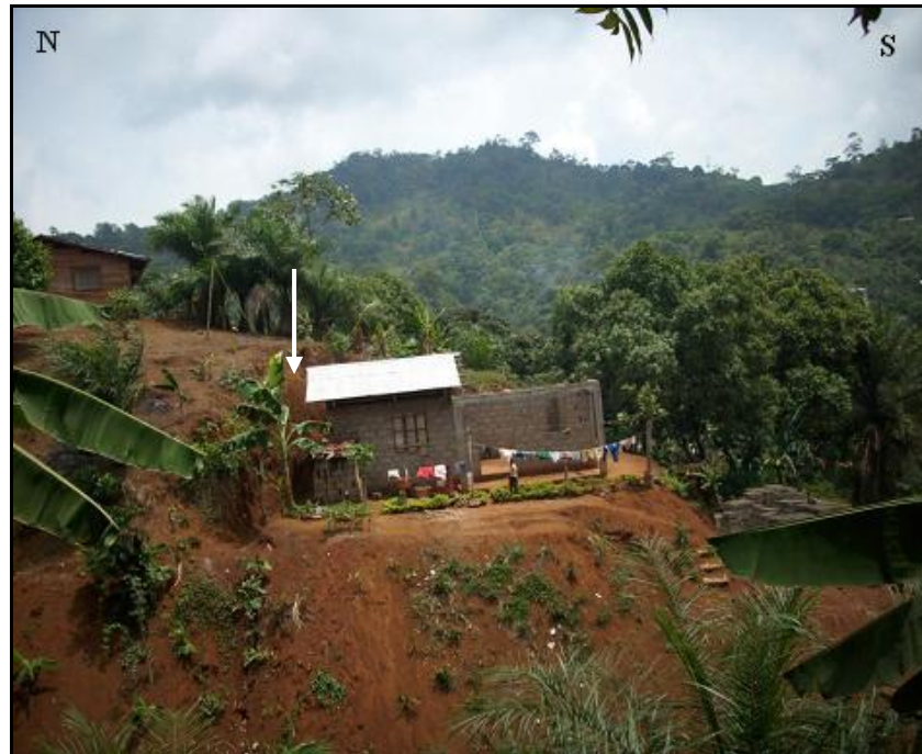
Fig. 2. 15. Close view of anarchical construction at Mabeta. Note terrace cut into slope to provide space for construction without any stabilization measure put in place. Excavated material piled down slope is a potential threat to down slope located buildings. White arrow indicates near slope created by construction works.
