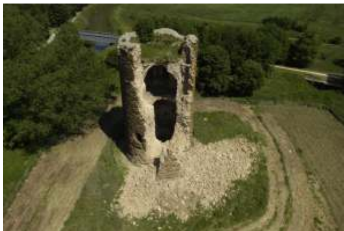
Figure 2: Maagdentoren at Zichem, an abandoned medieval four stage dungeon erected in the 14 th century, after its partial collapse in 2006 due to loading by roof breakdown, important soil deposit and long-lasting water infiltration. The structure has since been consolidated in its present form and protected against further infiltration. The present study deals with the standing walls not affected by the collapse.
