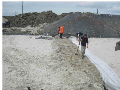
Figure 5. Installation of the geotextile before construction of the clay test dike.
