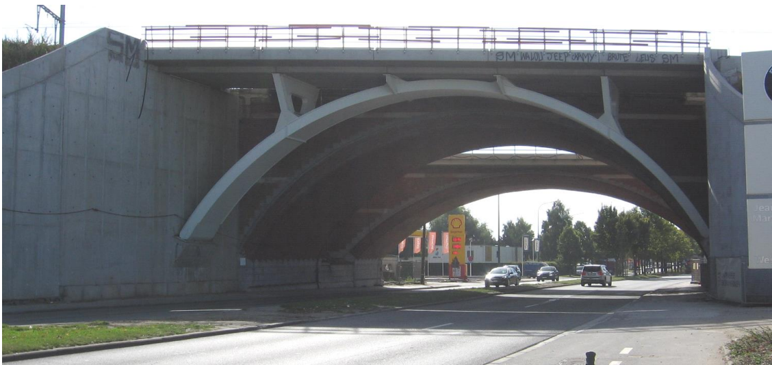
Figure 1. General view after erection of structure
