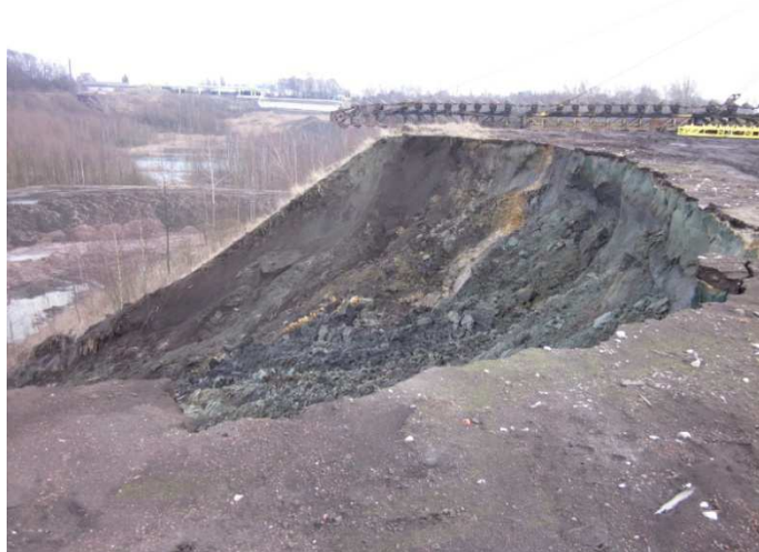
Fig. 6. Photo of the unstable zone after sliding
